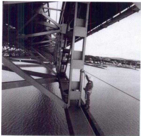
Figure 1 - HLL Installation under bridge
